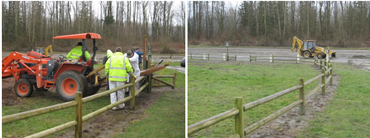
Flood damage repairs to Wiggly Field
