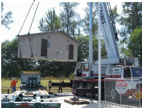
*Restroom section lifted into place by crane*
