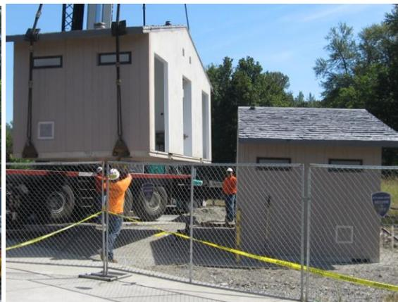
*Setting the two pre-fabricated restroom sections together*
