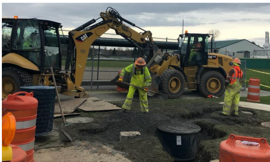
City utility crews installed a new duplex grinder pump system at Skykomish River Park.
