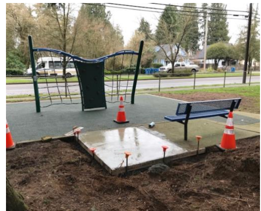
Left: Memorial bench installation at Lake Tye, Middle: Music ball foot room installation, Right: Concrete pad for GameNetic Game Console
