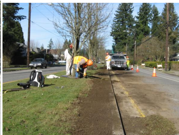
Landscape repair work @ Lewis St
