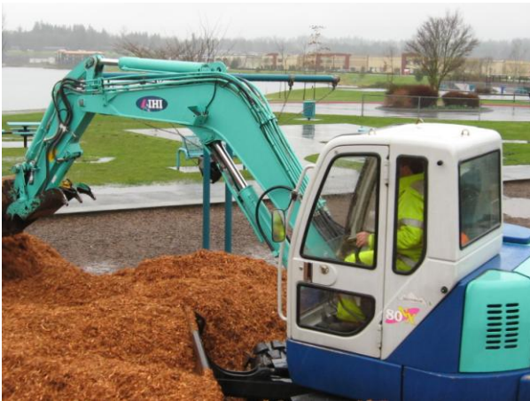
Eric Dexter operating trackhoe
